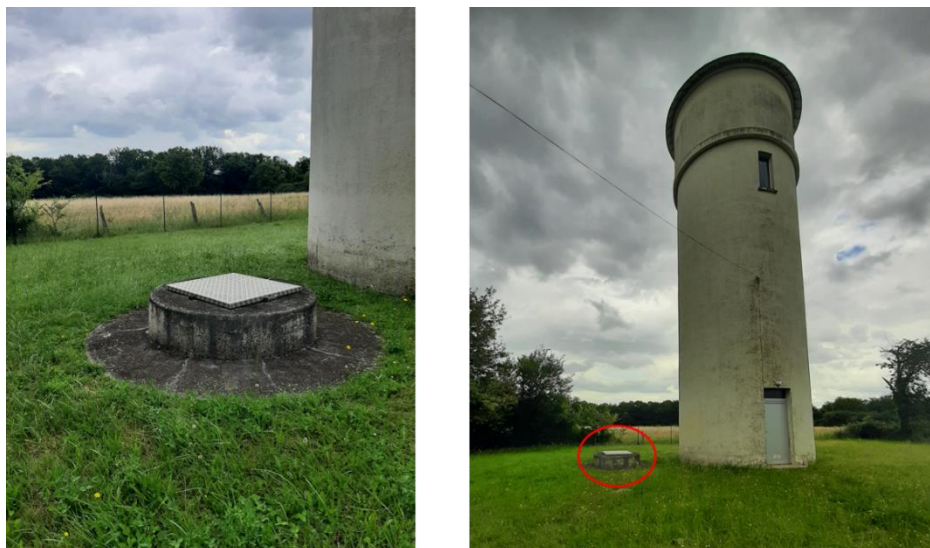
Figure 7 : Station de production forage Bel Air
